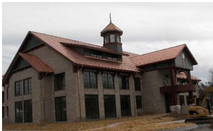
Fasig's new offices, still under construction
