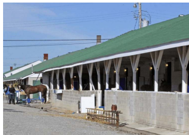
...and after renovation was completed Sept. 15 Reed Palmer photos
