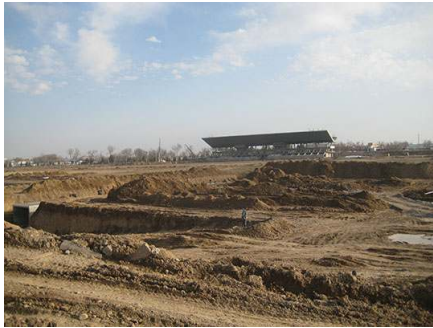
Construction at the track in Tashkent
