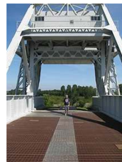
The original Pegasus Bridge is now part of the museum.
