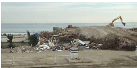
Across the street, crews begin the process of returning sand reclaimed from people's yards back to the beach
