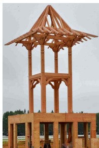
Construction of the Whitney viewing stand
